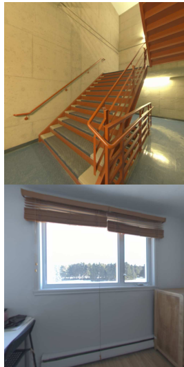
A concrete stairwell with orange railings leads up to a yellow door with a number 2 on it.
