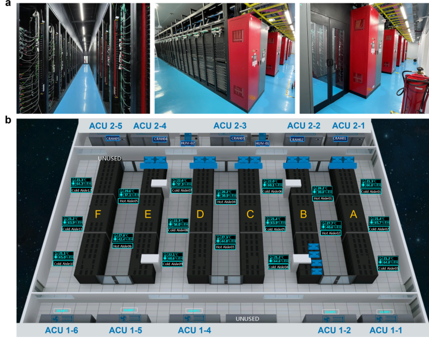
Figure 6: The photographs and layout illustration of the real-world commercial data center. a , Photographs of the interior of a server room, showcasing the hot aisle, cold aisle, and server racks from left to right. b , Overhead panoramic view of a server room, illustrating the spatial arrangement of all pertinent equipment.
