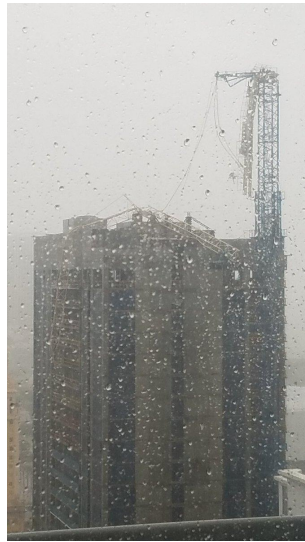
(c) A huge crane just collapsed on top of building in down town Miami
